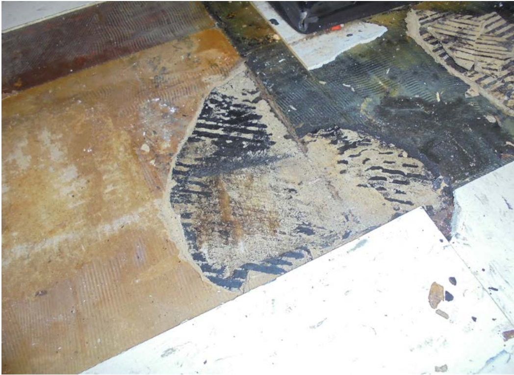
Photo 17: FT layers, 12" over 9" with black mastic, Room #33
