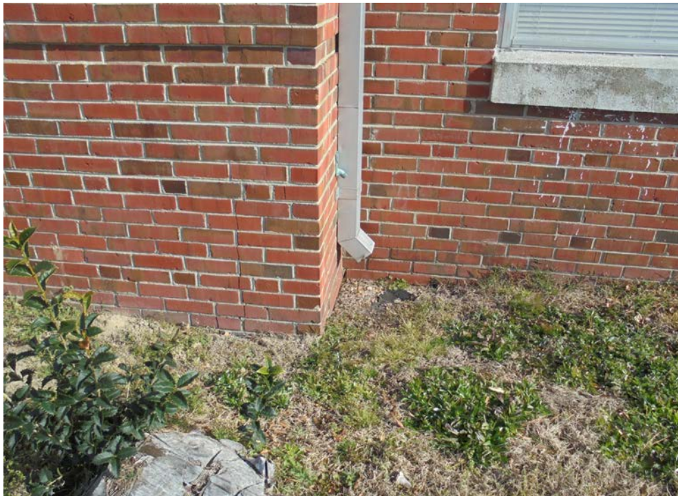
Photo 2: Poor drainage away from structure.
