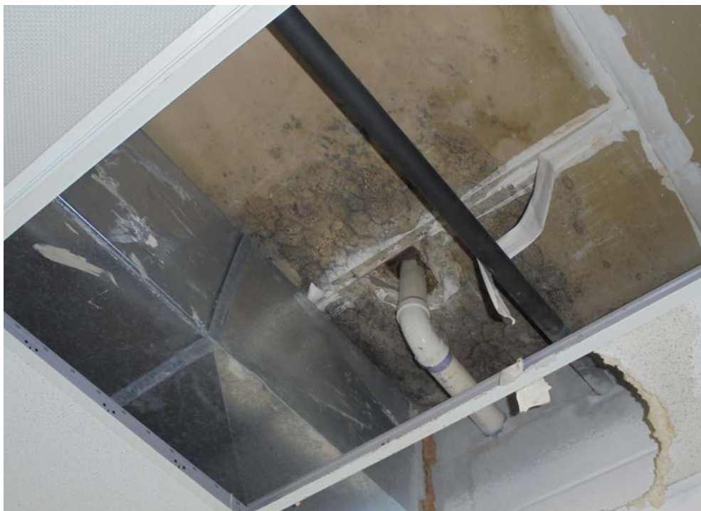
Photo 12: VMG on ceiling drywall, Room #5.
