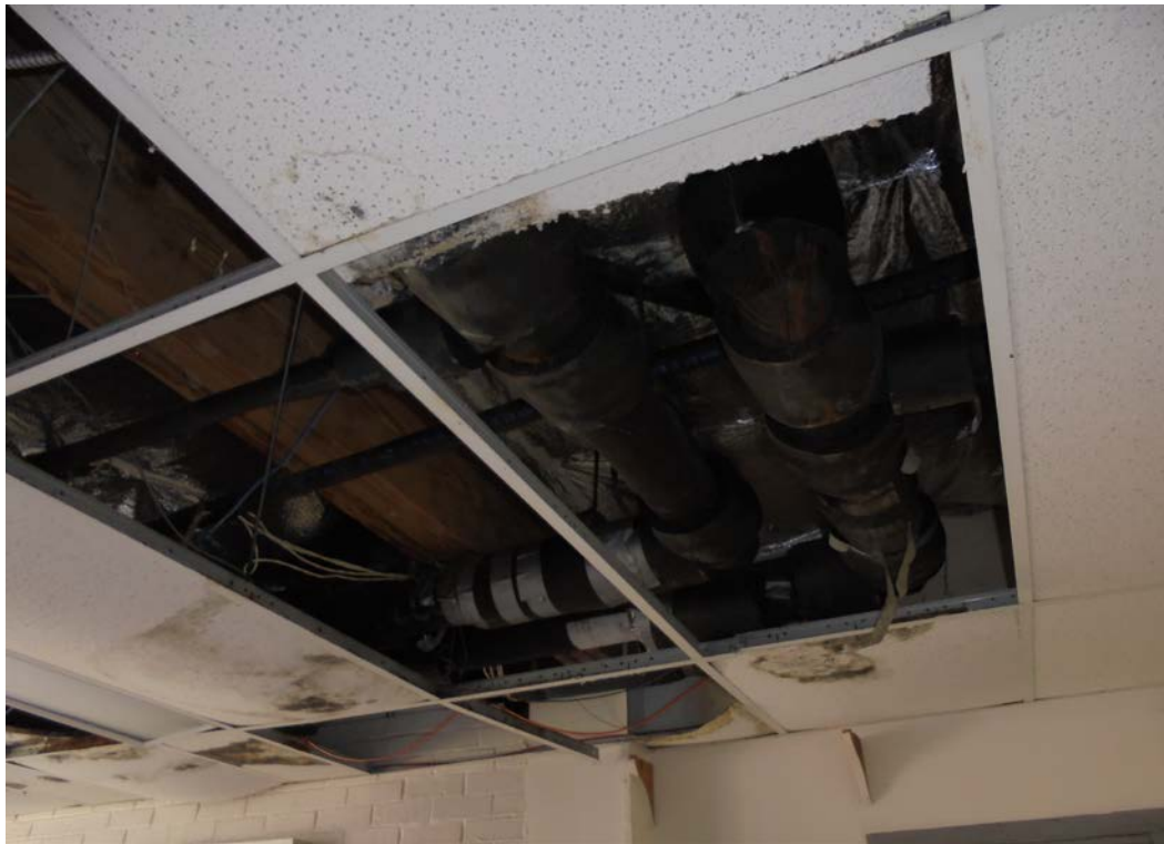
Photo 15: Overhead TSI on mechanical lines, 80s 90s transition area.
