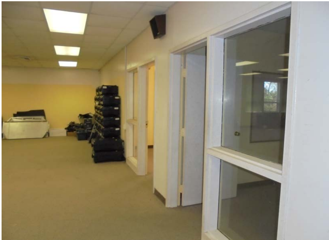
Photo 13: Media Center, VMG on surfaces and area had unpleasant mildew odor.
