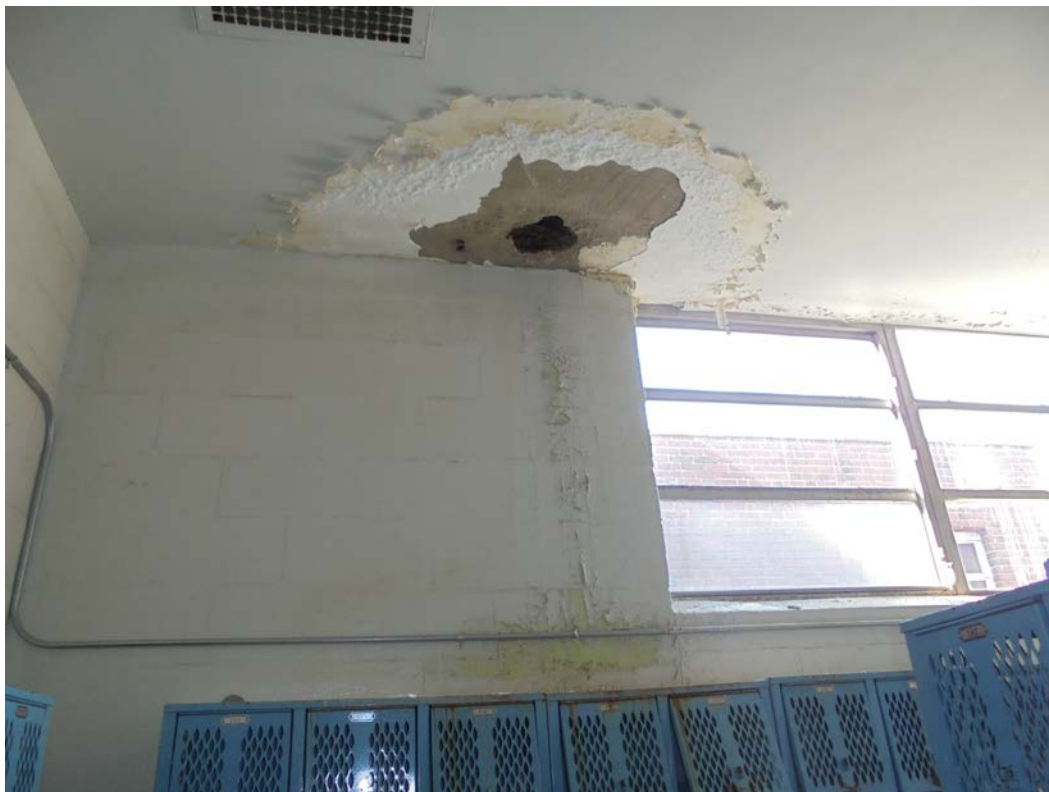
Photo 5: Moisture damage, boy's locker room.
