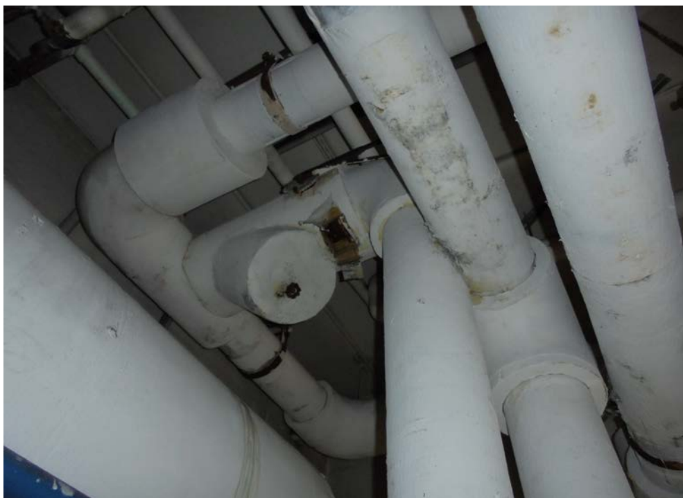
Photo 6: VMG on mechanical room TSI.
