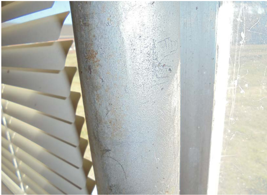
Photo 19: LBP on support poles Room #34
