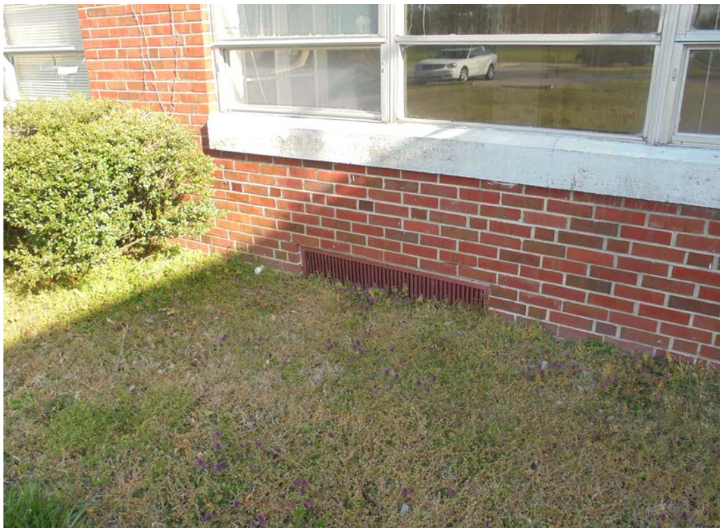
Photo 3: Vegetation and poor drainage from AHU fresh air intake.
