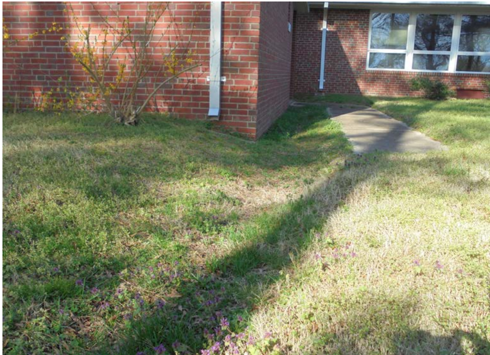
Photo 4: Ground view appears to flow back towards building and swale.
