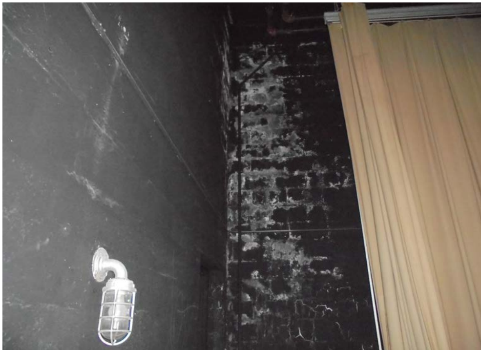
Photo 14: Auditorium stage, efflorescence .
