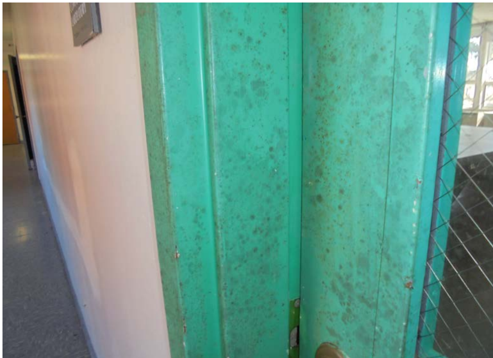
Photo 10: VMG on metal painted surfaces 1980s wing.
