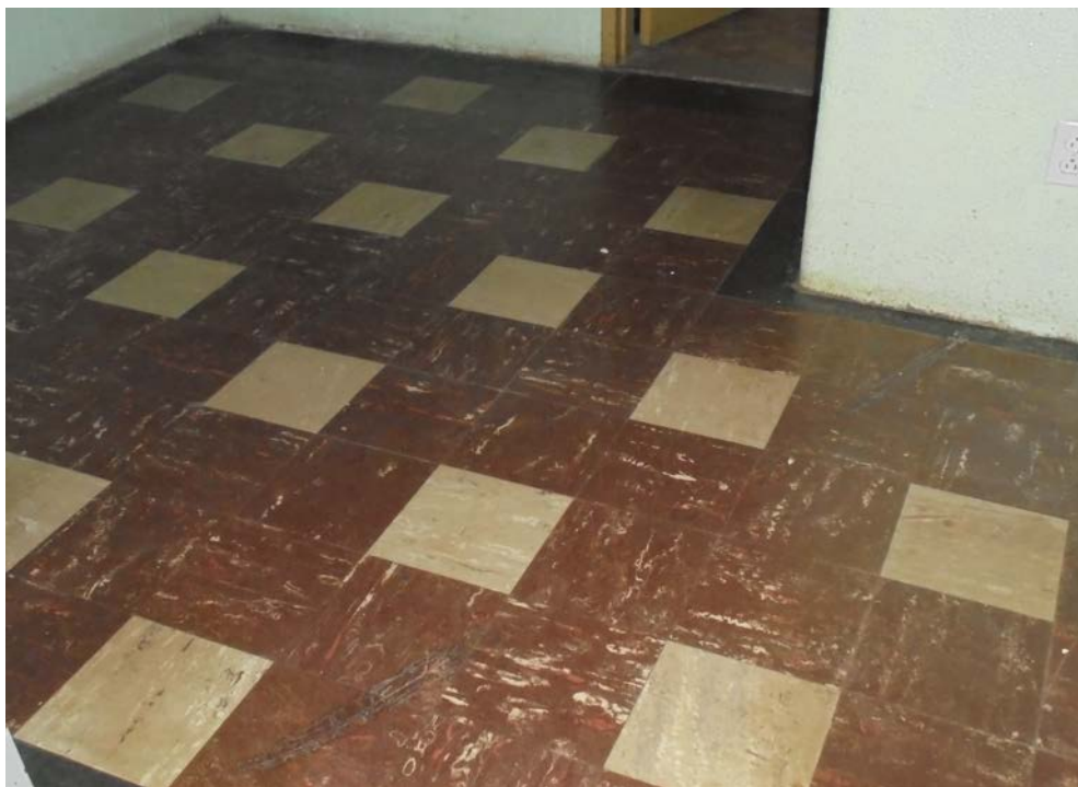
Photo 16: Typical 9"x9" FT, restroom/locker area at Gym.
