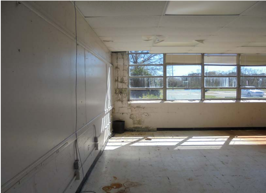
Photo 7: VMG contamination and moisture damage in Room #23.
