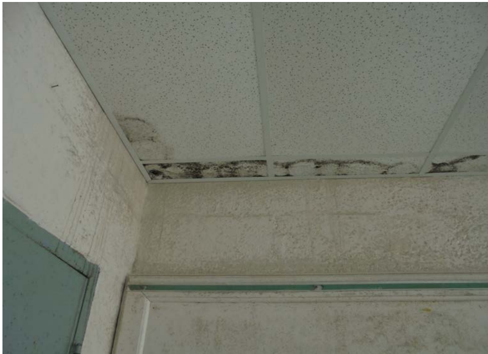
Photo 8: VMG contamination Room #25.
