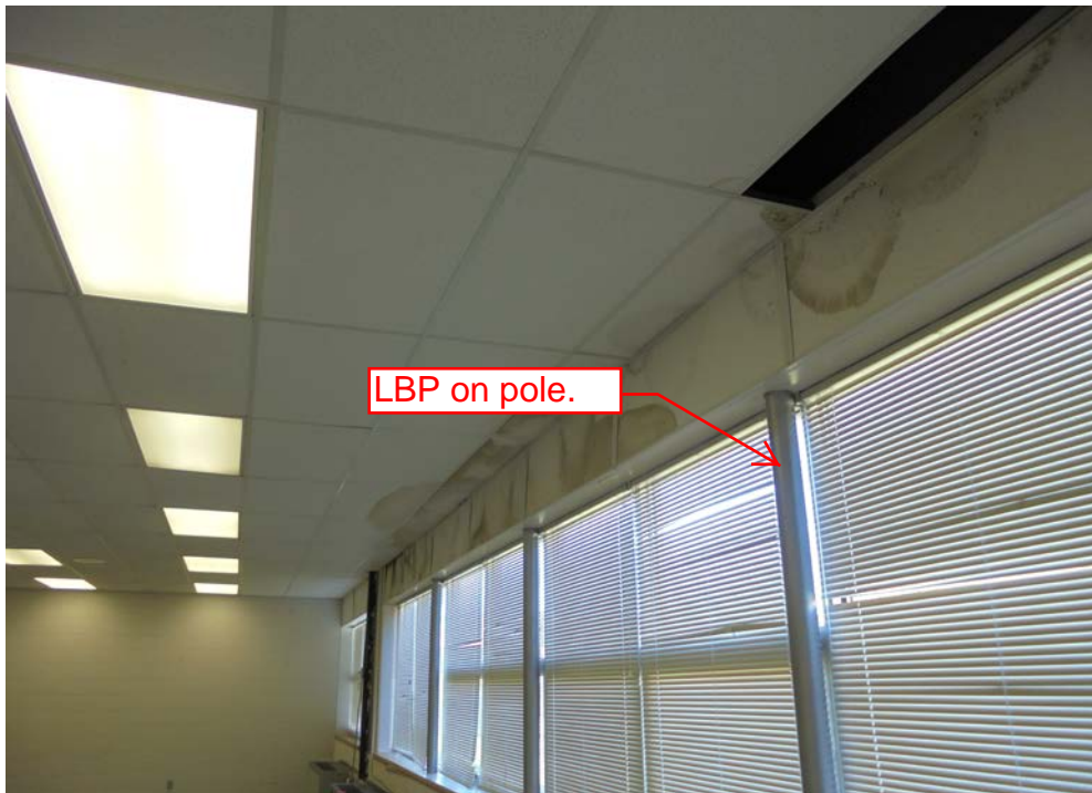
Photo 20: Broad view of LBP and pole location.
