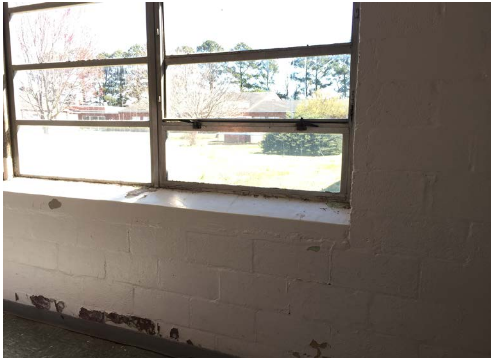
Photo 18: Old framed windows with AB window glaze, hall at Gym.
