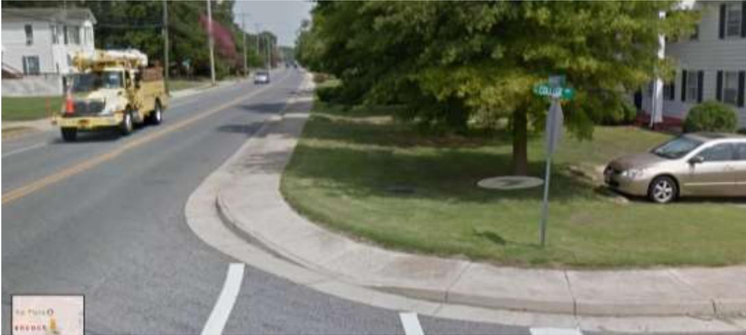
3. Non-functional - less than 3 feet wide, missing ramps and/or flares, utility poles in sidewalk, broken, heaved, etc. Any one of these conditions qualifies the sidewalk for this category. This view is Justis Street in Onancock.
