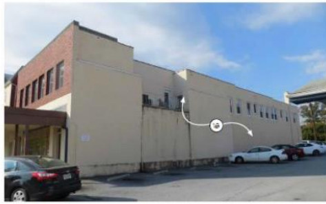
EXISTING SIDE FACADE
