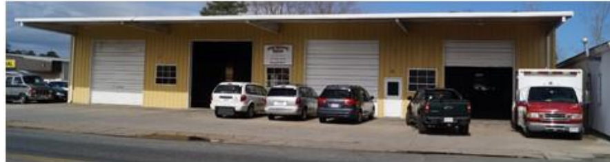
P29 – Shore Transport Services Storage, 24345 Bennett St. Economic Blight: No; Physical Blight: Yes but structurally sound
