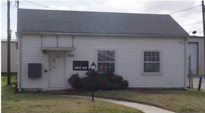
P49 – Verizon Building, 24332 Adelaide St. Economic Blight: No; Physical Blight: No
