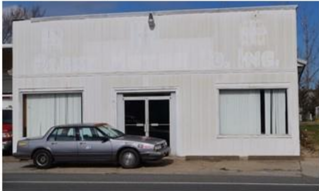
P28 – Shore Transport Services Storage, 24355 Bennett St. Economic Blight: No; Physical Blight: Yes but structurally sound
