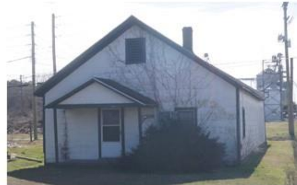
P10 – Vacant Structure, 24248 Bennett St.
