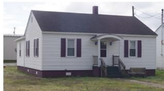
P48 – Private Residence, 24338 Adelaide St. Economic Blight: No; Physical Blight: No
