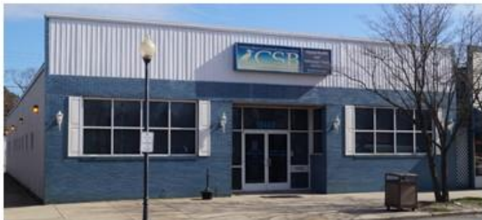
P53 – Eastern Shore Community Services Board, 18469 Dunne Ave. Economic Blight: No; Physical Blight: Yes but structurally sound
