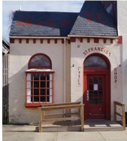
P56 – Former Bayside Rehab, 18477 Dunne Ave. Economic Blight: Yes; Physical Blight: Yes but structurally sound
