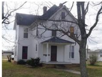
P47 – Private Residence, 24344 Adelaide St. Economic Blight: No; Physical Blight: No
