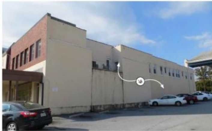
EXISTING SIDE FACADE
