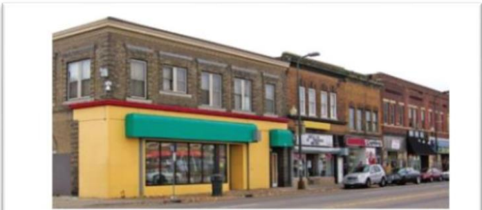
BEFORE Covering brick with another material, like the yellow boards in this photograph, is discouraged.
