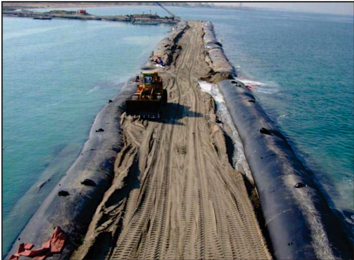
Figure 5-8. Geotextile dike example (from the TenCate Geosynthetics website). This geotextile is used for illustrative purposes only; VIMS does not provide recommendations for any particular company.
