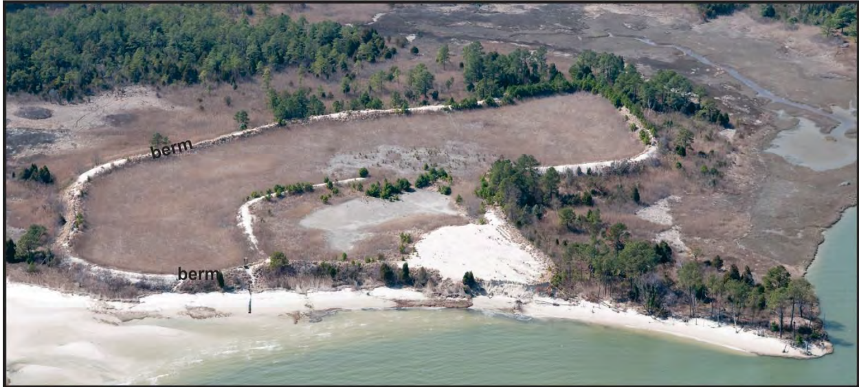
Figure 3-2. Inactive confined disposal area at Winter Harbor, Mathews County, VA. Much of the site has become vegetated. The front corner berm/dike is being eroded. Photo: 7 March 2010 Shoreline Studies Program, VIMS.
