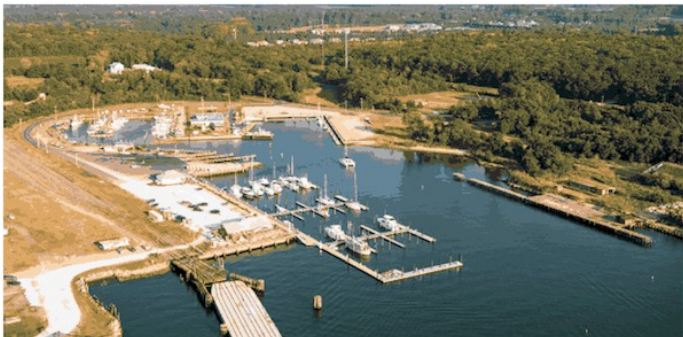
Southeasterly aerial view of the Cape Charles Town Harbor. The facility is a designated Harbor of Refuge that serves a variety of commercial, recreational, and industrial users. Credit: Cape Charles Wave.
