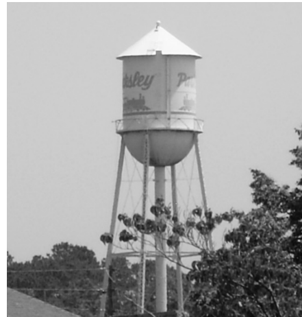
Figure 3: Parksley Water Tower. Photo by Curt Smith
