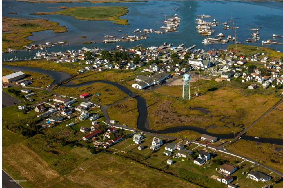
Figure 6: Aerial view of West Ridge, West Ridge Creek, Main Ridge, and the Mail Channel, featuring the water tower west of the Swain Memorial United Methodist Church and one of the main cemeteries. Photo ©2016 Gordon Campbell/At Altitude Gallery
