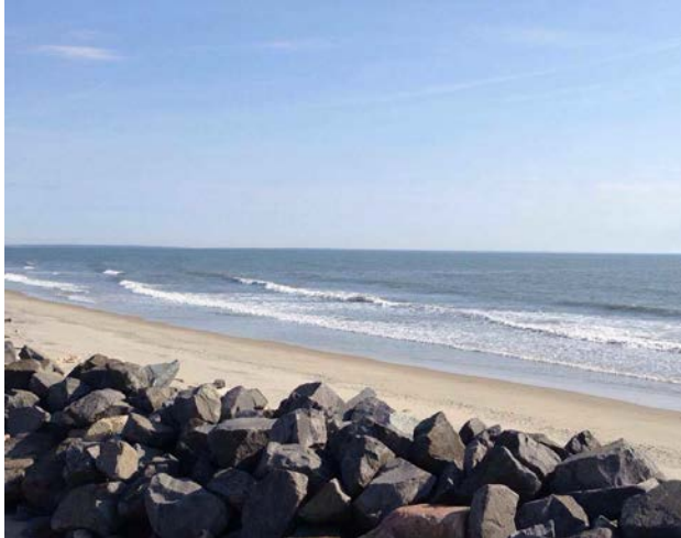
Figure 8: Revetment at the beach of Wallops Flight Facility. Photo Credit: NASA
