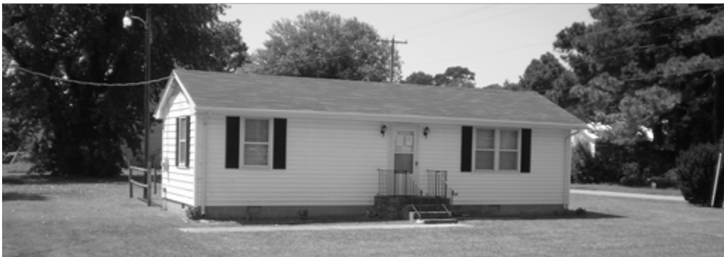
Figure 4: The Keller Town Office is at risk from storm water flooding and wind damage. Photo by Curt Smith
