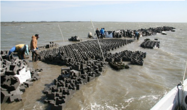
Figure 11: Oyster Reef under Construction Photo Credit: © Bowdoin Lusk/ The Nature Conservancy. Used with permission.
