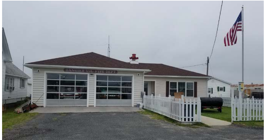
Figure 3: Tangier Firehouse. Photo by Shannon Alexander
