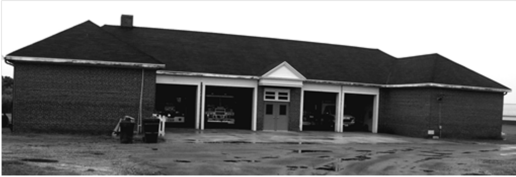
Figure 4 : Saxis' firehouse and Town office are located in a flood zone. Photo by Elaine Meil.
