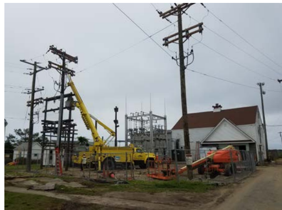
Figure 7: Electric substation. Photo by Shannon Alexander
