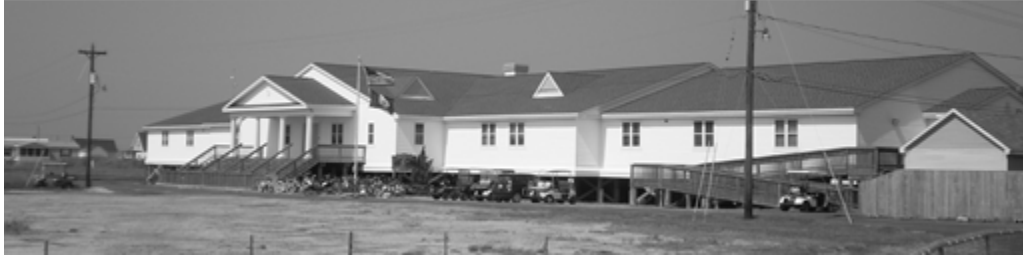
Figure 8: The Tangier Combined School was elevated in 2006 to mitigate flood damages. Photo by Curt Smith
