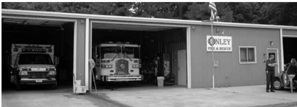
Figure 2: Onley Volunteer Fire and Rescue Department. Photo by Ann Devletian, 2003-04
