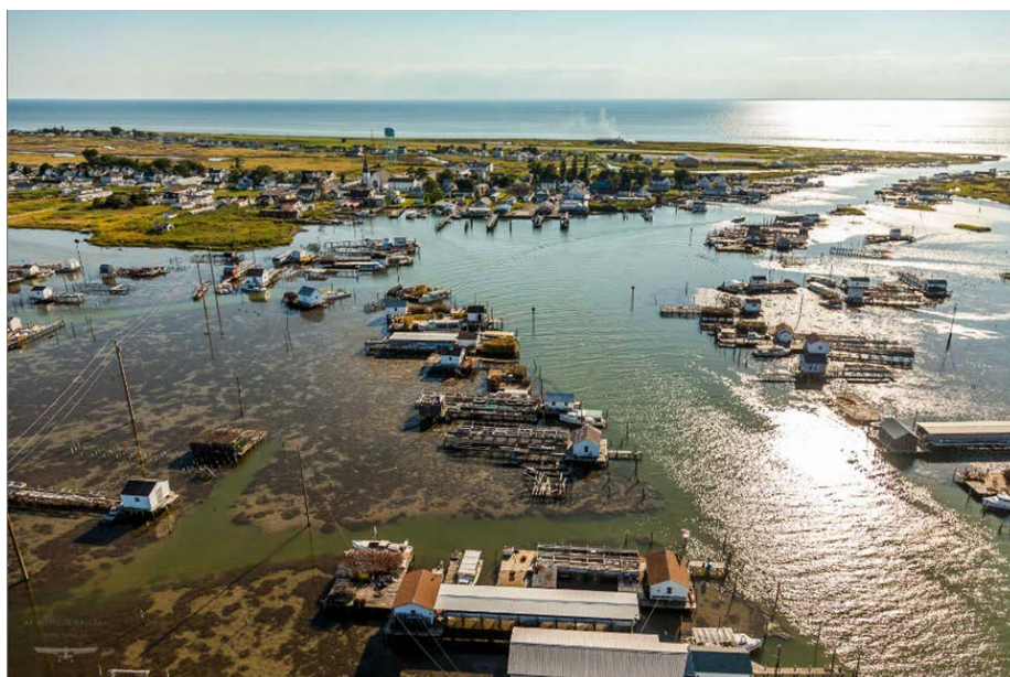
Figure 13: Crab and waterman houses on Tangier can easily be damaged during storms, such as Hurricane Isabel. Photo ©2016 Gordon Campbell/At Altitude Gallery
