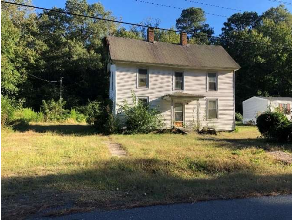
Figure 11: There are several structures in poor condition. A sagging roofline indicates serious structural issues that require expensive renovations. In these instances, demolition and replacement may be more affordable.
