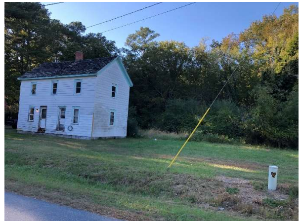
Figure 14: Many homes had wear and tear with siding. Others had more serious issues, especially with roofing. In this example, the roof shingles are deteriorating.
