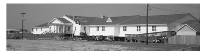
Figure 8: The Tangier Combined School was elevated in 2006 to mitigate flood damages. Photo by Curt Smith
