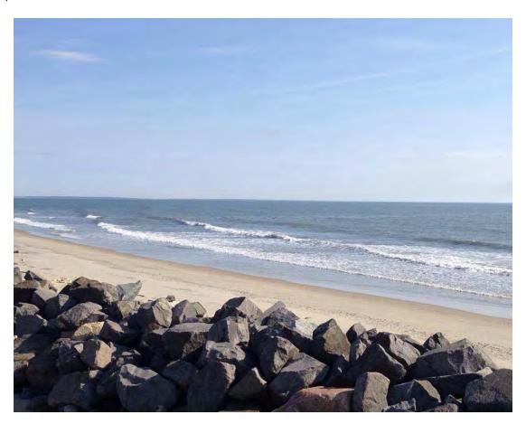
Figure 7: Revetment at the beach of Wallops Flight Facility. Photo Credit: NASA
