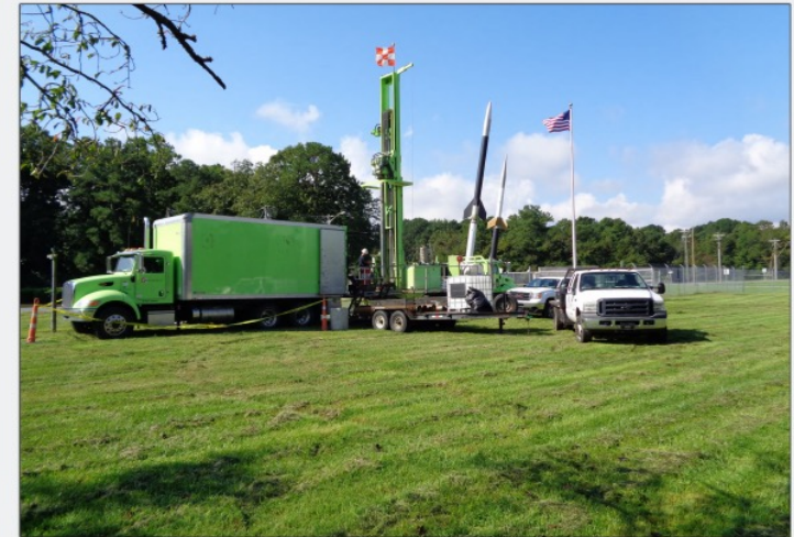
Installation of PFAS perimeter monitoring well via roto-sonic drilling
