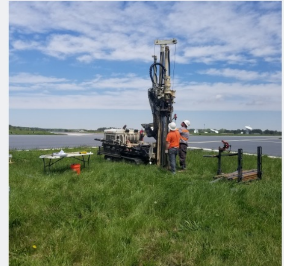
Soil and groundwater sample collection
