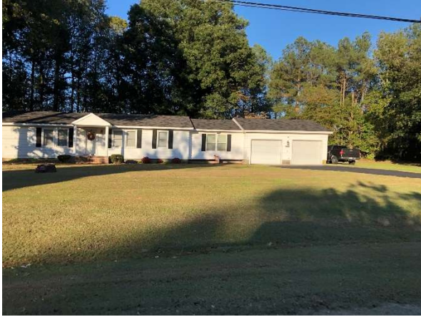
Figure 15: Most residential structures are in "fair" to "good" condition. This single-family home is one example of a structure in good condition.
