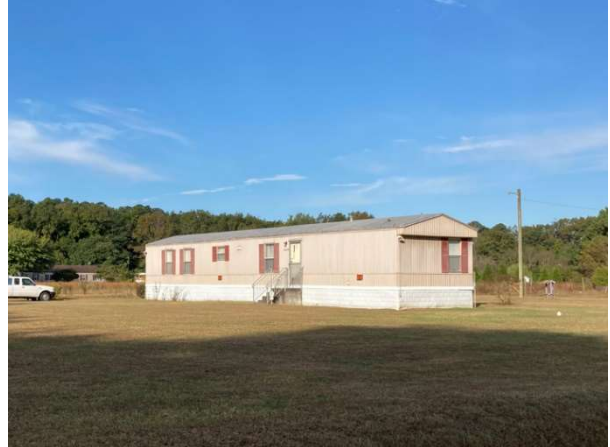
Figure 8: The area includes a large number of mobile homes ranging from newer models in good condition to older models in need of improvement or replacement.
