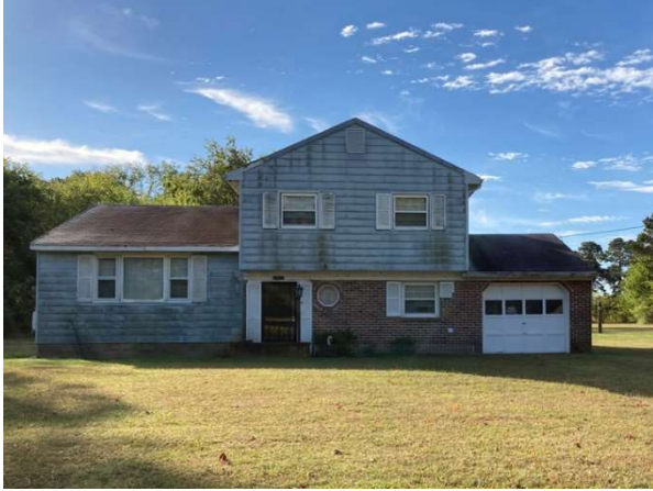
Figure 7: Many observed units had maintenance needs, including siding, window, and roof repairs that may help them remain occupied dwellings.
